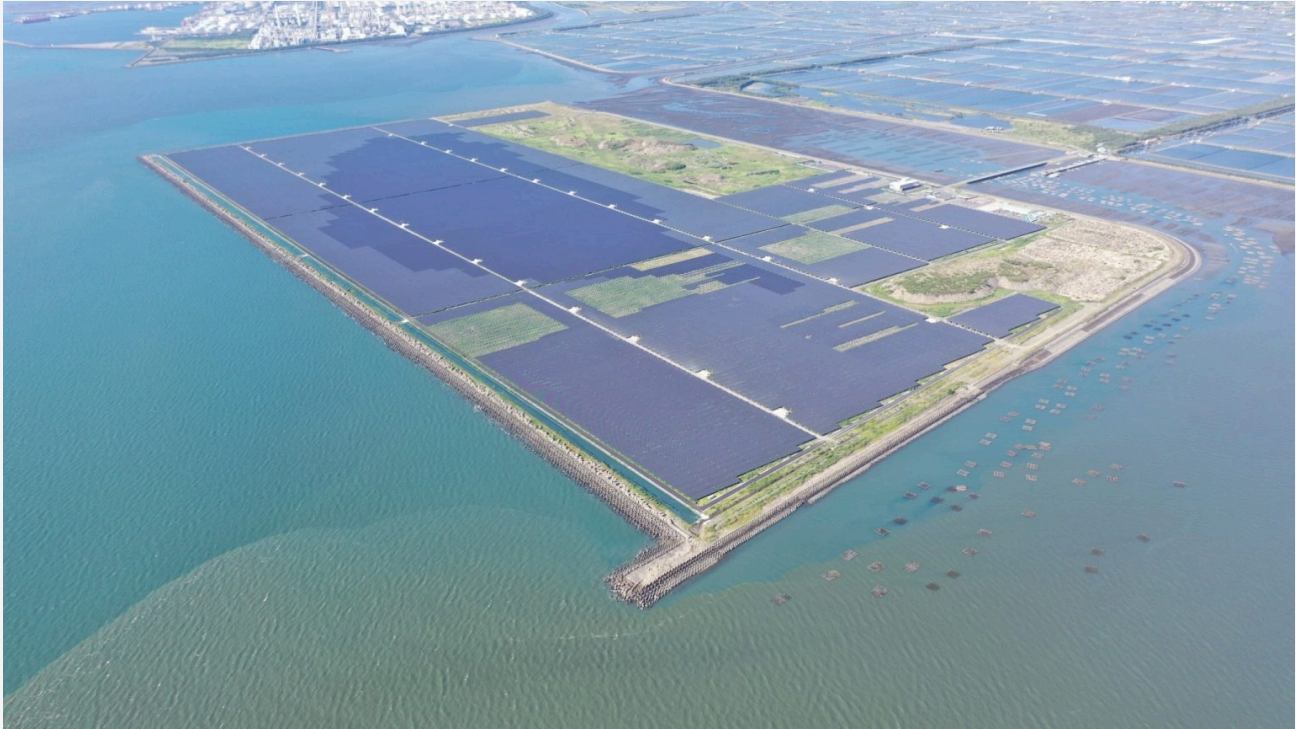
The Yunlin E2 Solar Project currently under construction in Taiwan.
